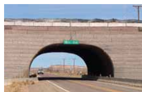
Corrugated Structural Plate: Cost effective and quickly installed, with range of shapes to accommodate various span lengths.
