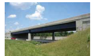
Plate Girder: Fabricated as parallel flange, tapered or haunched girders.
