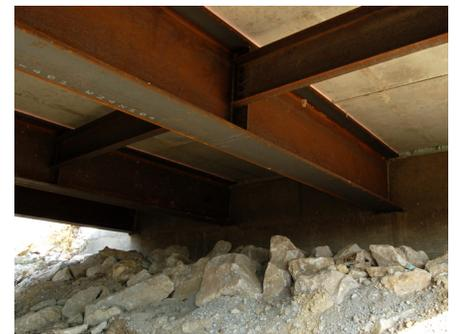
Mann noted that the lower price per square-foot for the steel bridge was driven by the fact that the steel girders were less than half the price of the slab girders. Crane costs also created some of the savings.
