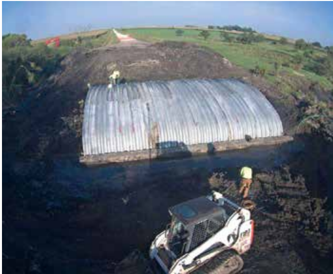
Figure 4. The 200 th Street Bridge project during construction.
