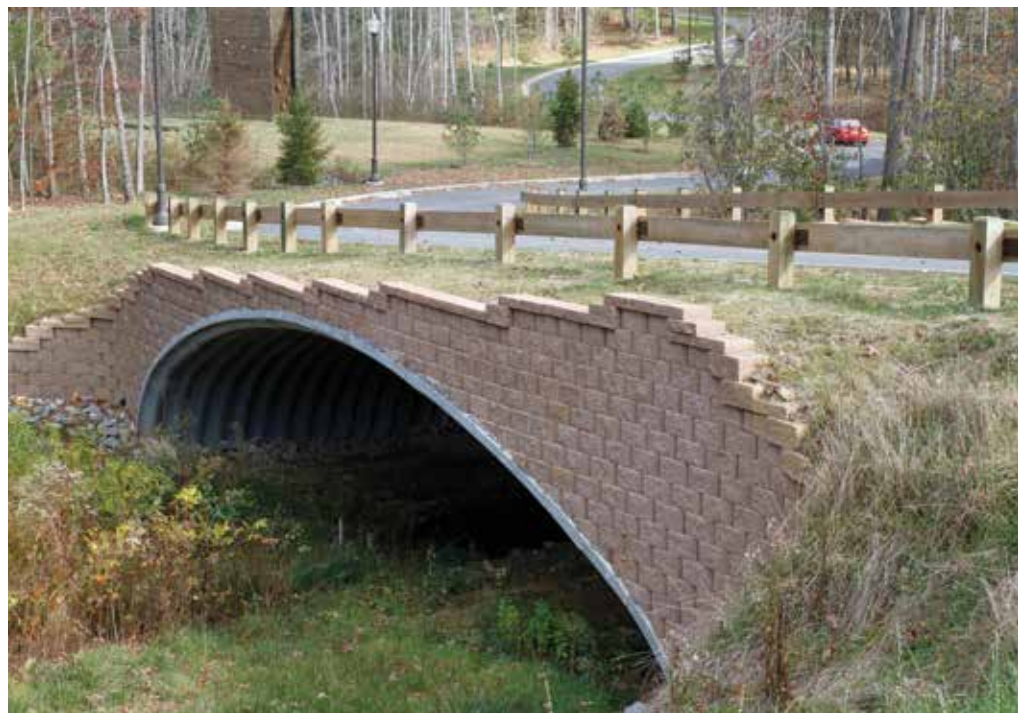
Figure 1. A steel buried bridge.
