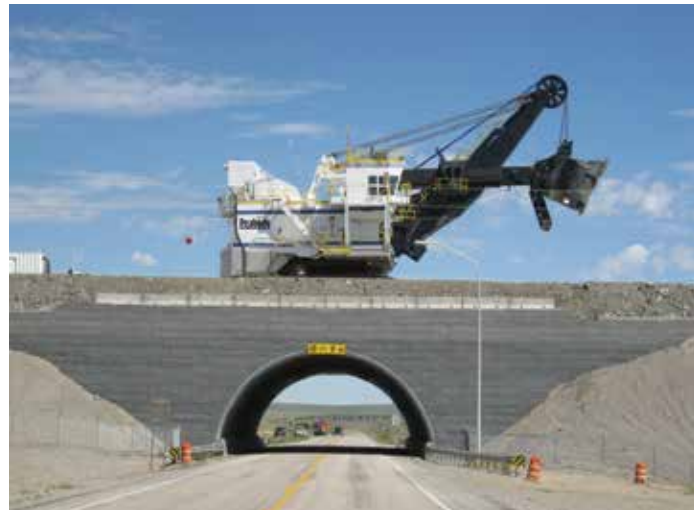
Figure 3. Steel buried bridges can be designed to support very heavy loads.
