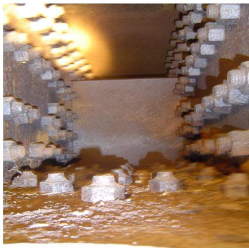
Fig. 6. Corrosion inside open truss member
