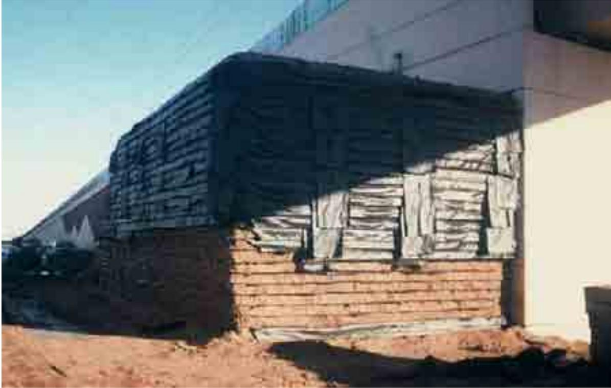
**Figure 8. Photo. Internally supported GRS structure.**
