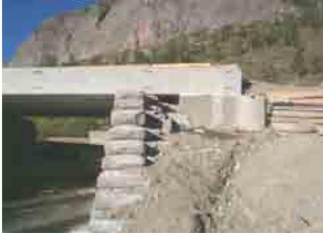
**Figure 32. Photo. GRS abutment behind historic stone abutment.**
