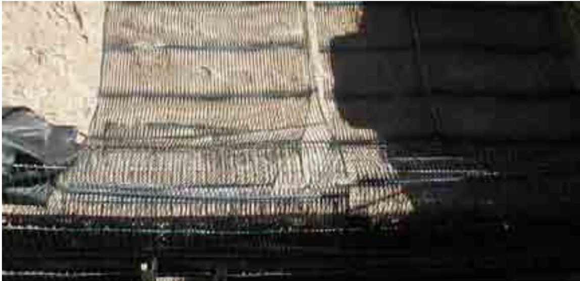
**Figure 4. Photo. MSE extensible reinforcement (geogrid).**
