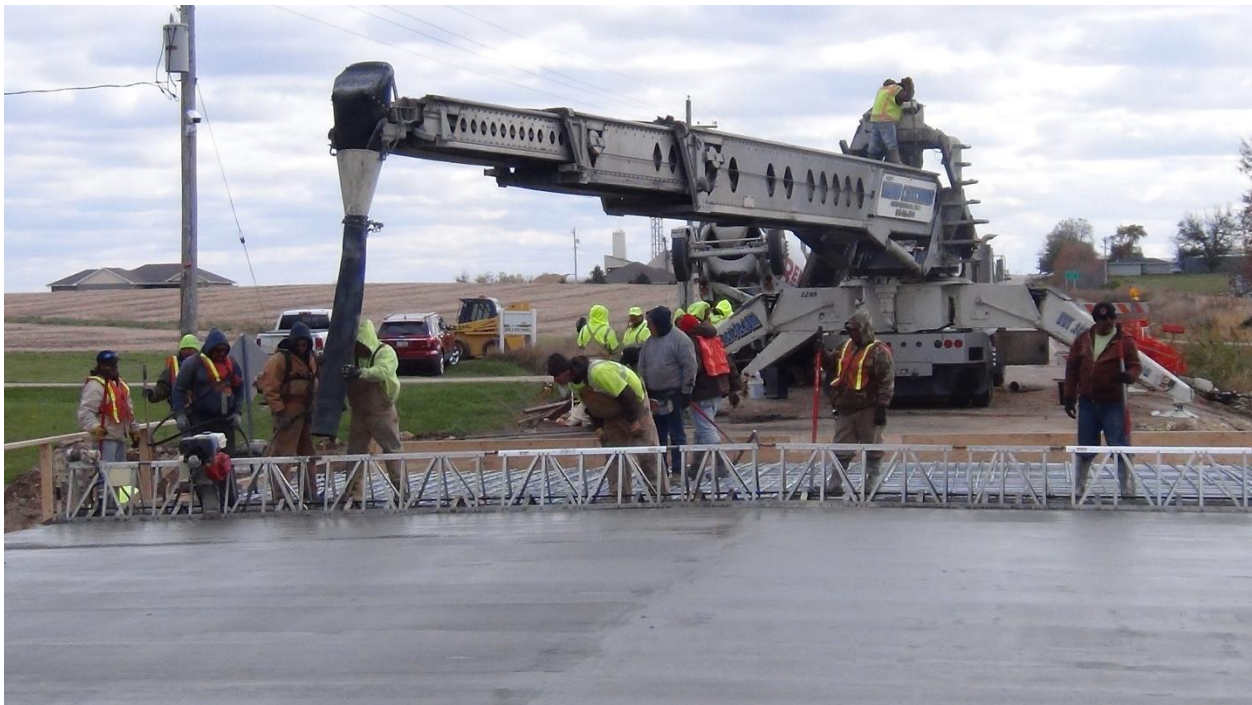
Figure 5.5: Placement of Concrete Deck
