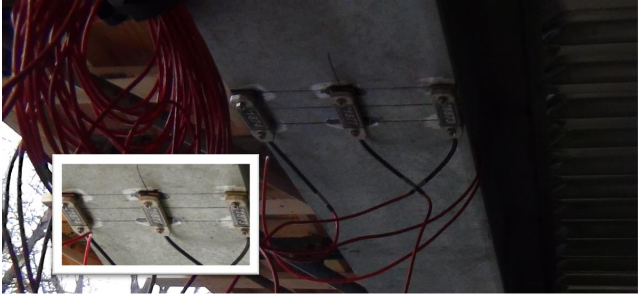
Figure 5.3: Bottom Flange Gage Locations (10' from Abutment Face)
