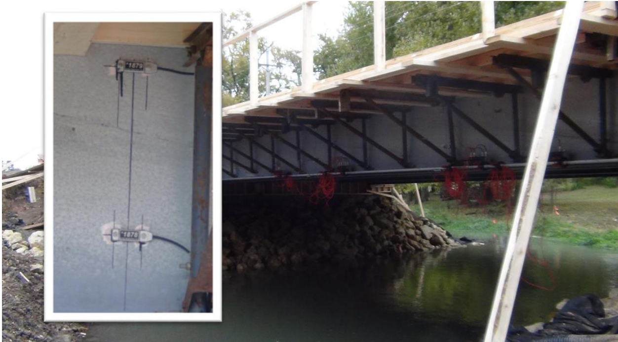
Figure 5.4: Web Gage Locations (10' from Abutment Face, Exterior Gages Visible)
