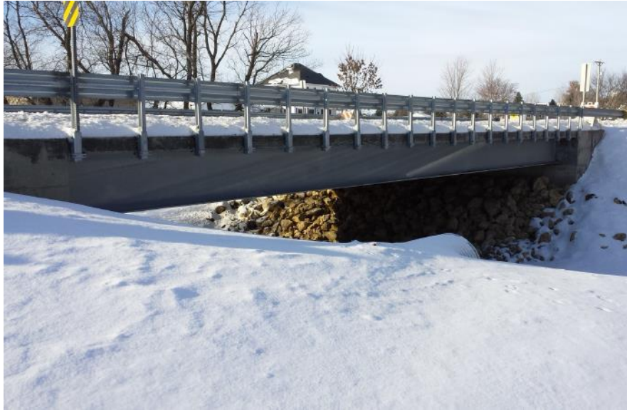
Figure 3.2: Newly-Completed Jesup South Bridge, Constructed in 2013 (Case Study)
