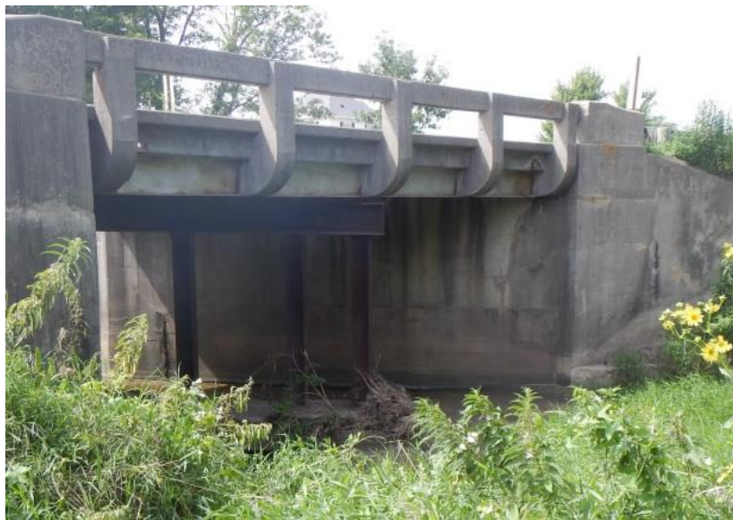
Figure 3.1: Old Jesup South Bridge, Constructed in 1947 (Case Study)
