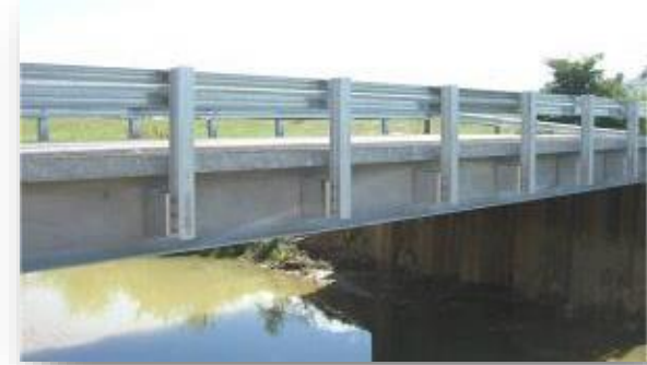
Rolled Beam Shape
