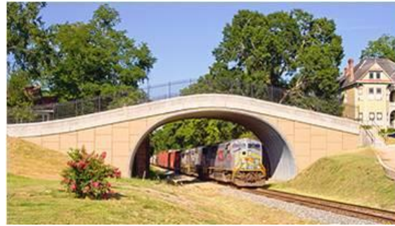
Corrugated Steel Plate (Buried Steel Bridge)
