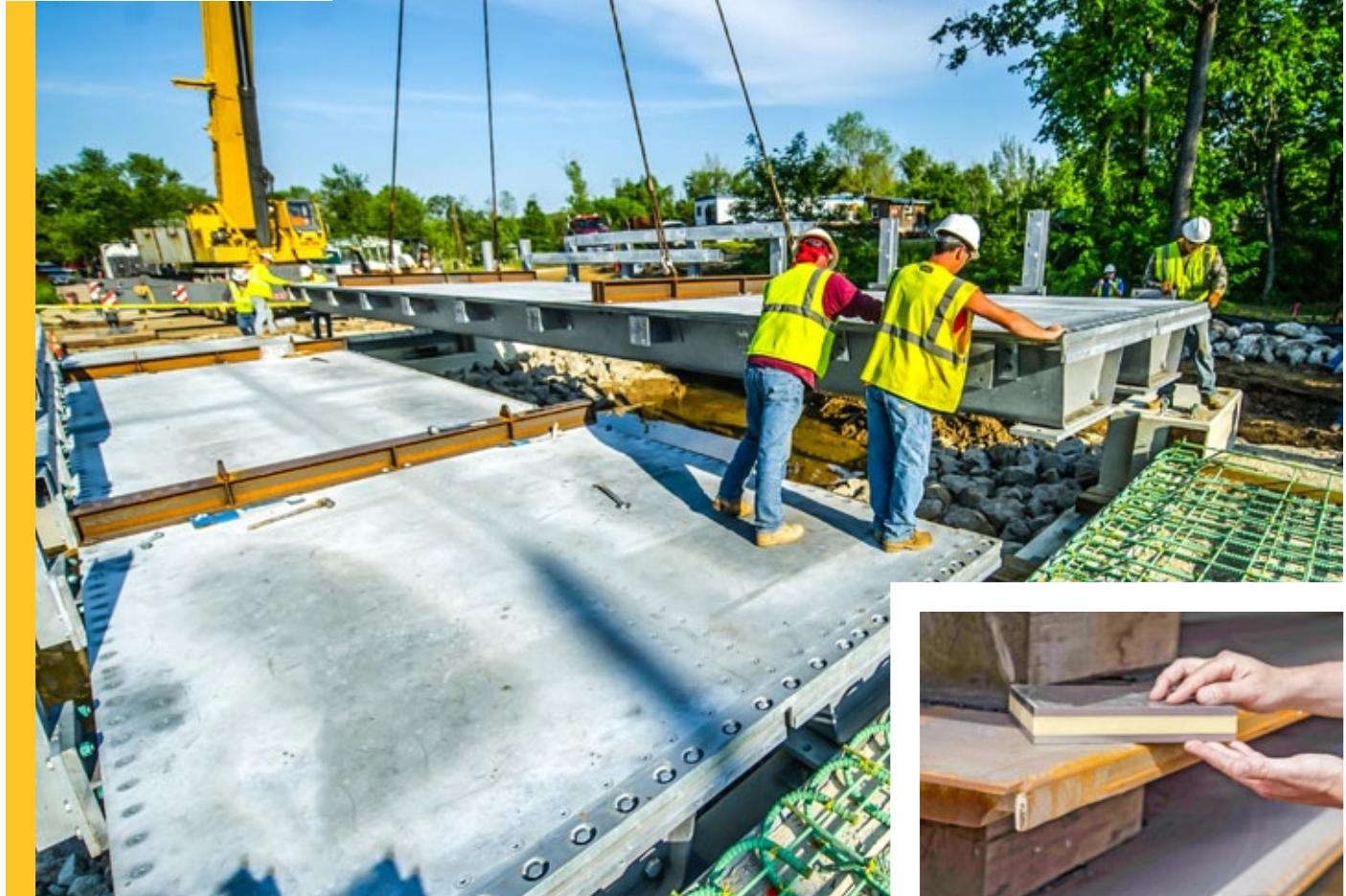
→ The Sandwich Plate System (SPS®) is a structural composite material used for bridge decks that is up to 70% lighter than reinforced concrete. A high precision component manufactured offsite, makes it easy and quick to install.
