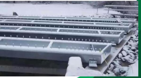
Henry Road Bridge, Mercer County, PA Field Assembly - Composite Precast Deck Panels
