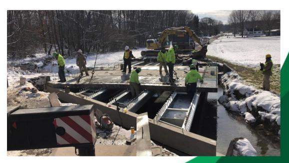
Henry Road Bridge, Mercer County, PA Field Assembly - Composite Grouted Shear Pockets
