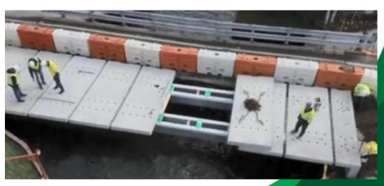
Henry Road Bridge, Mercer County, PA Field Assembly - Composite PBTGs no Deck
