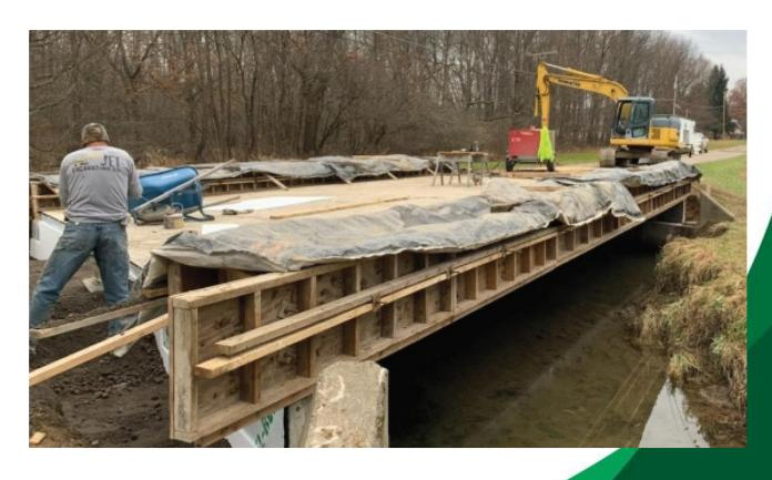
Henry Road Bridge, Mercer County, PA Field Assembly - Composite Completed Bridge
