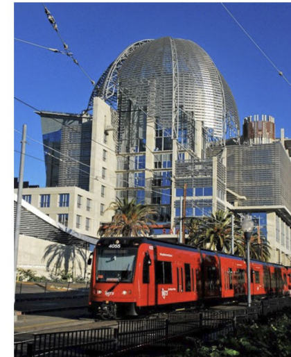
The San Diego Central Library façade and dome utilizes hot-dip galvanized hot-rolled sections, plate, and hollow structural steel sections.
