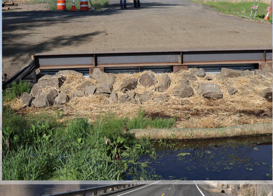
Modular Components Delivered And set on abutments.
