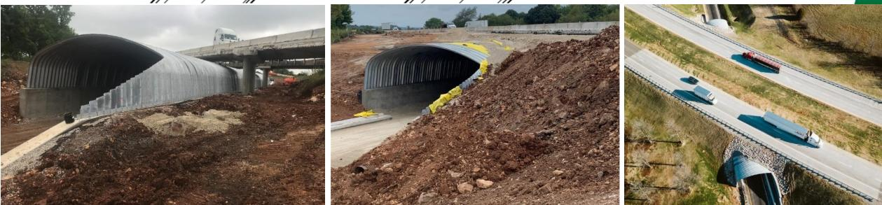
Customized layouts & end treatments to accommodate site configurations: CR1147 – step beveled ends to match fill slope
