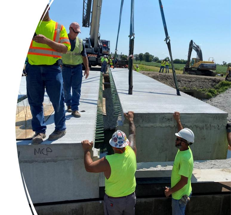
Beams are Pinned 8" Closure Pour Between Beams
