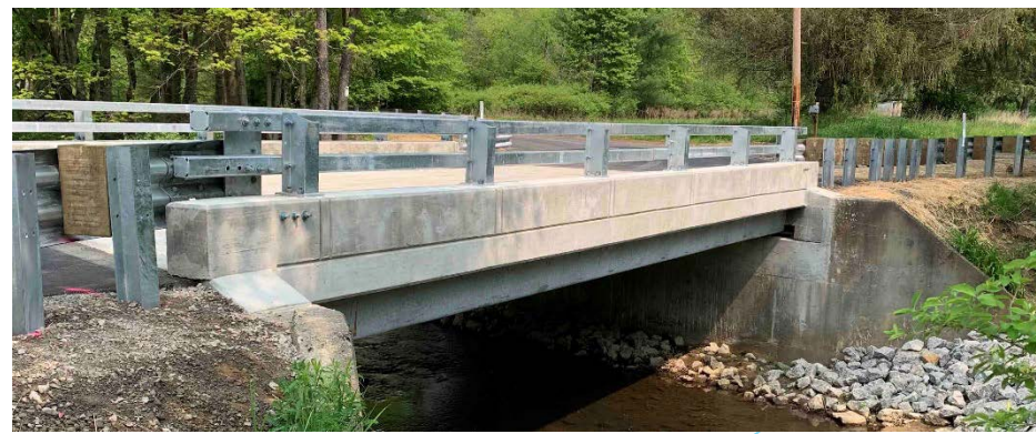
MERCER COUNTY, PA – 40' SPAN – 20° SKEW PennDOT LOADING - PHL-93
