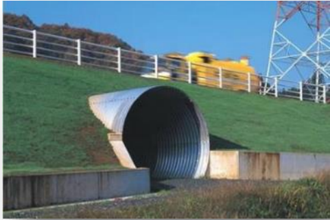
Corrugated Steel Pipe (Buried Steel Bridge)
