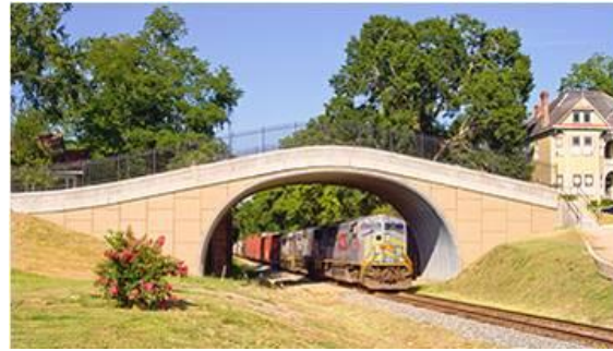
Corrugated Steel Plate (Buried Steel Bridge)
