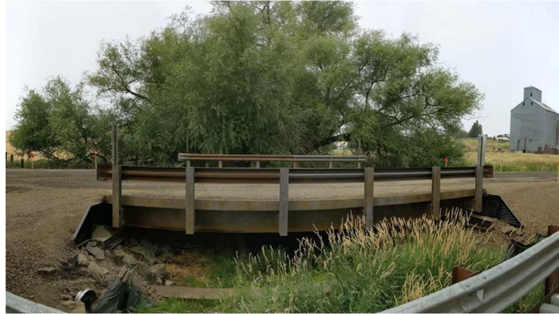
New Bridge 30 ft long / 28 ft wide TrueNorth Modular Steel Bridge Installed by County Crew
