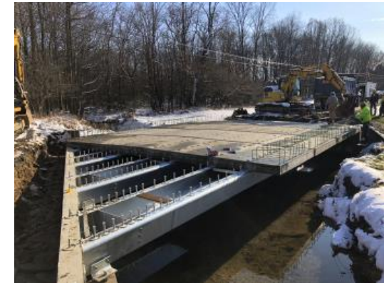
Press-Brake Tub Girder
