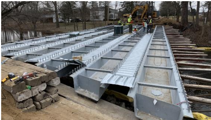
Press-Brake-Formed Tub Girders
