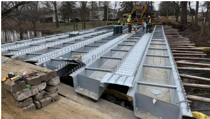
Press-Brake-Formed Tub Girders
