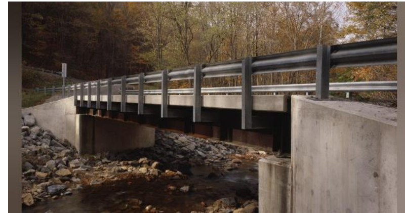
Rolled Beam & Plate Girders
