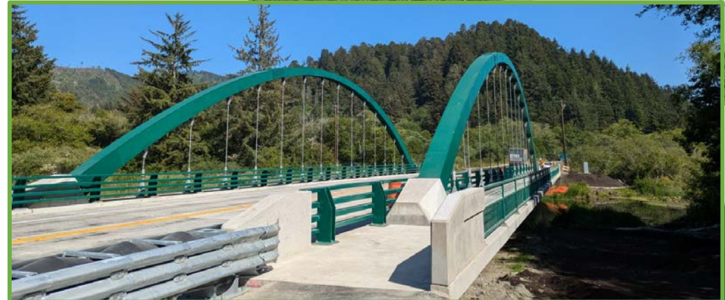
Panther Creek Bridge, Klamath, CA | 2024
