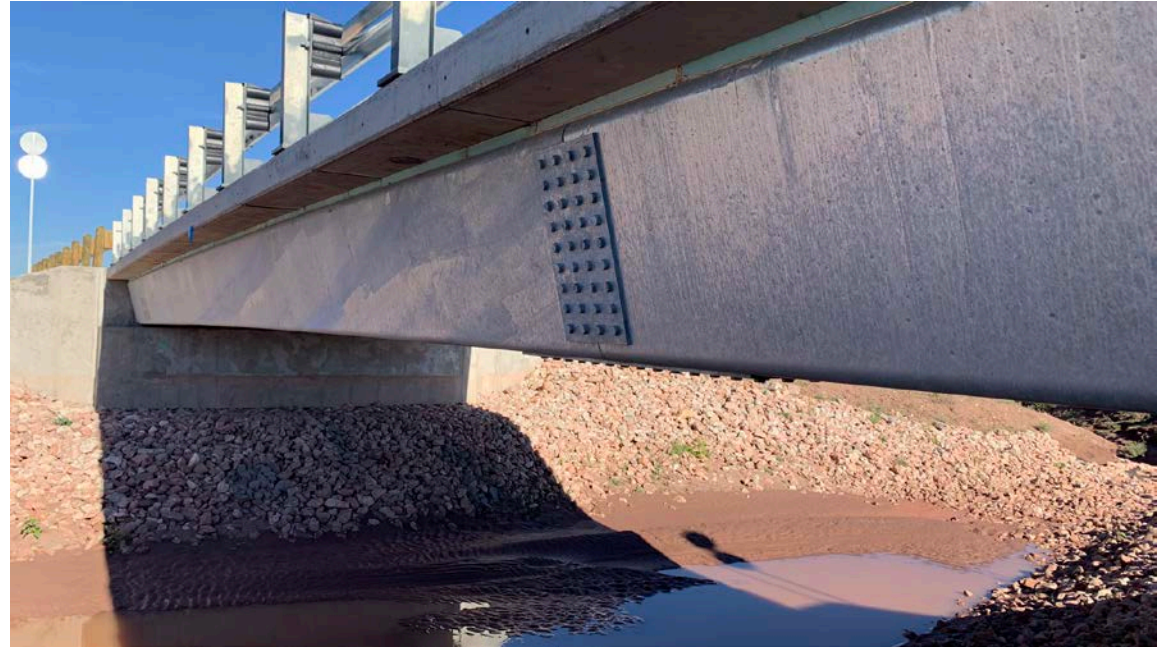
USACE Fort Wingate Bridge Replacement Gallup, NM | 2022 52 tons – Press-brake-formed steel tub girder: 8 beams weighing 12,600 lbs. each
