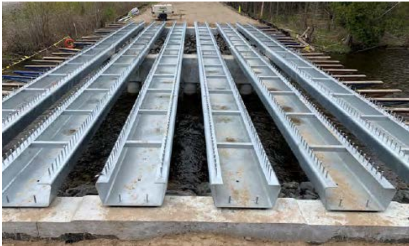
PBFTG STANDARD TUB GIRDER CROSS SECTION
