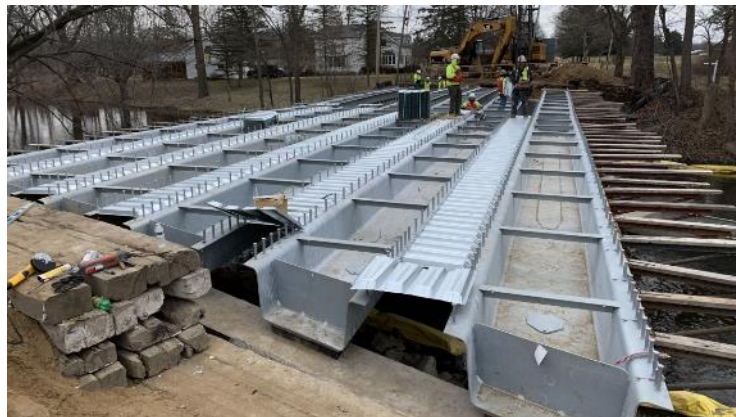
Press-Brake-Formed Tub Girders
