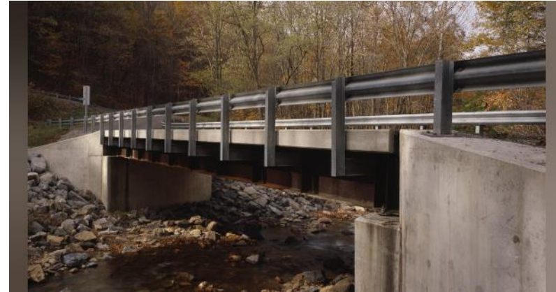
Rolled Beam & Plate Girders
