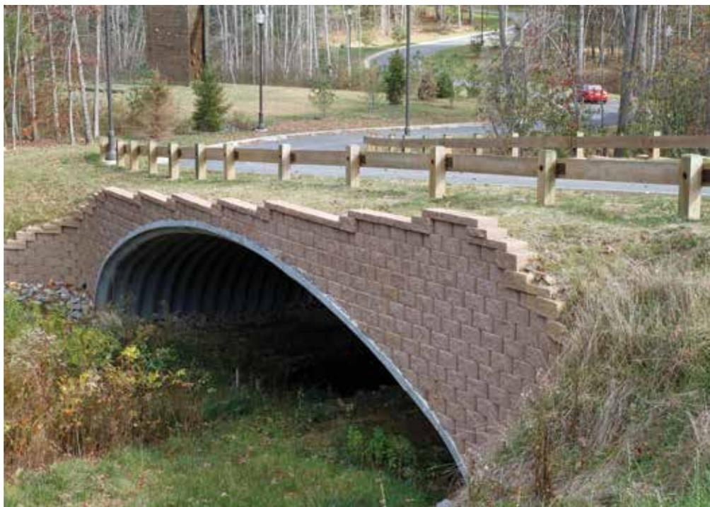
*Figure 1. A steel buried bridge.*
