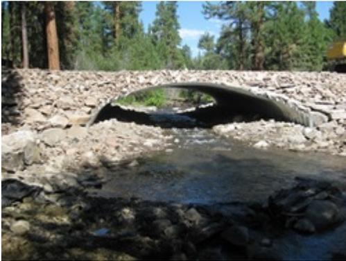
resistivity values outside of the recommended limits, galvanized steel will be unsuitable, but that's not the case. Since a select granular material will be in contact with the structure, the site soils should not have major impact on service life. If contact with soils outside of the recommended pH and resistivity range is unavoidable, secondary coatings can be applied or other measures taken as a precaution.
