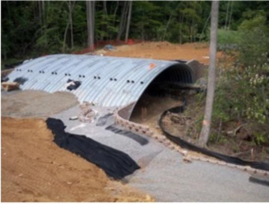
design and a budget cost for a buried bridge structure and compare that to the cost of a different bridge system. That's a mistake. They need to look at everything involved with constructing that project, not just the cost of the structure by itself. When site costs and foundation costs are factored into the total cost equation, the steel option can be significantly less expensive than a precast structure, sometimes on the
