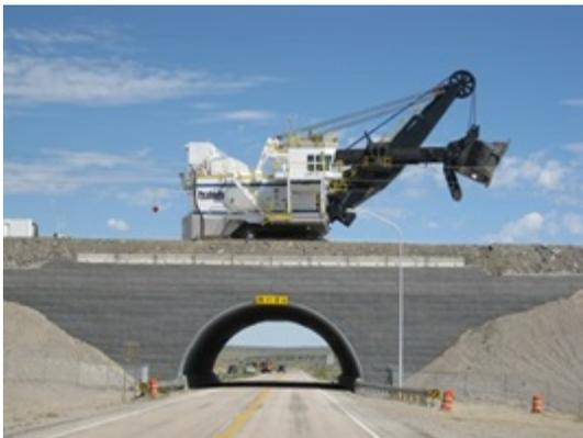
There are also many cases where buried bridges can carry heavier loads than traditional bridges because of the benefits of spreading vehicle loads through the fill. Buried bridges do not require abutments; and unless foundation soil conditions are poor, do not typically require deep foundations. Because of this, little differential movement or settlement between the buried bridge and adjacent embankments can be expected. This
